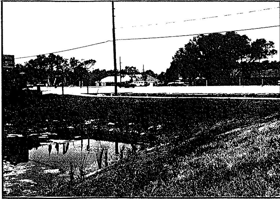
SITE C5A West Side of U.S. 19
