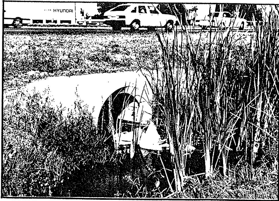
SITE A-1B East of U.S. 19 Looking West
