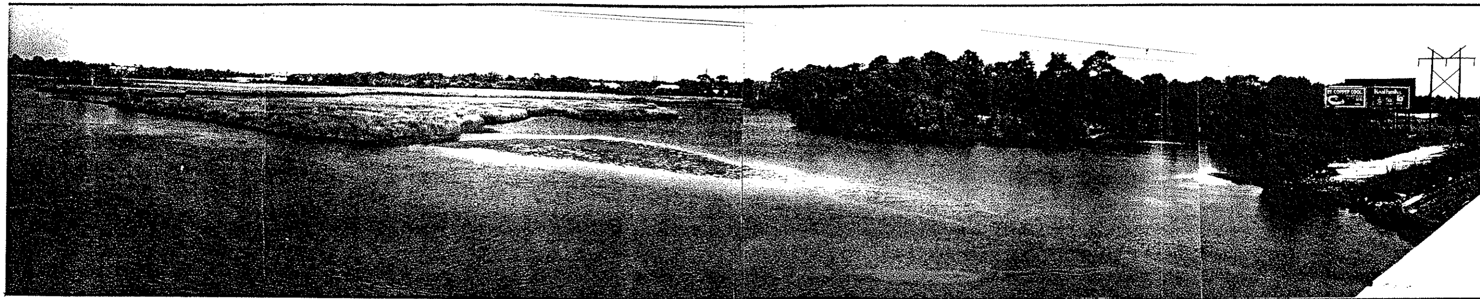
ANCLOTE RIVER - East Of U.S. 19 Looking Upstream
